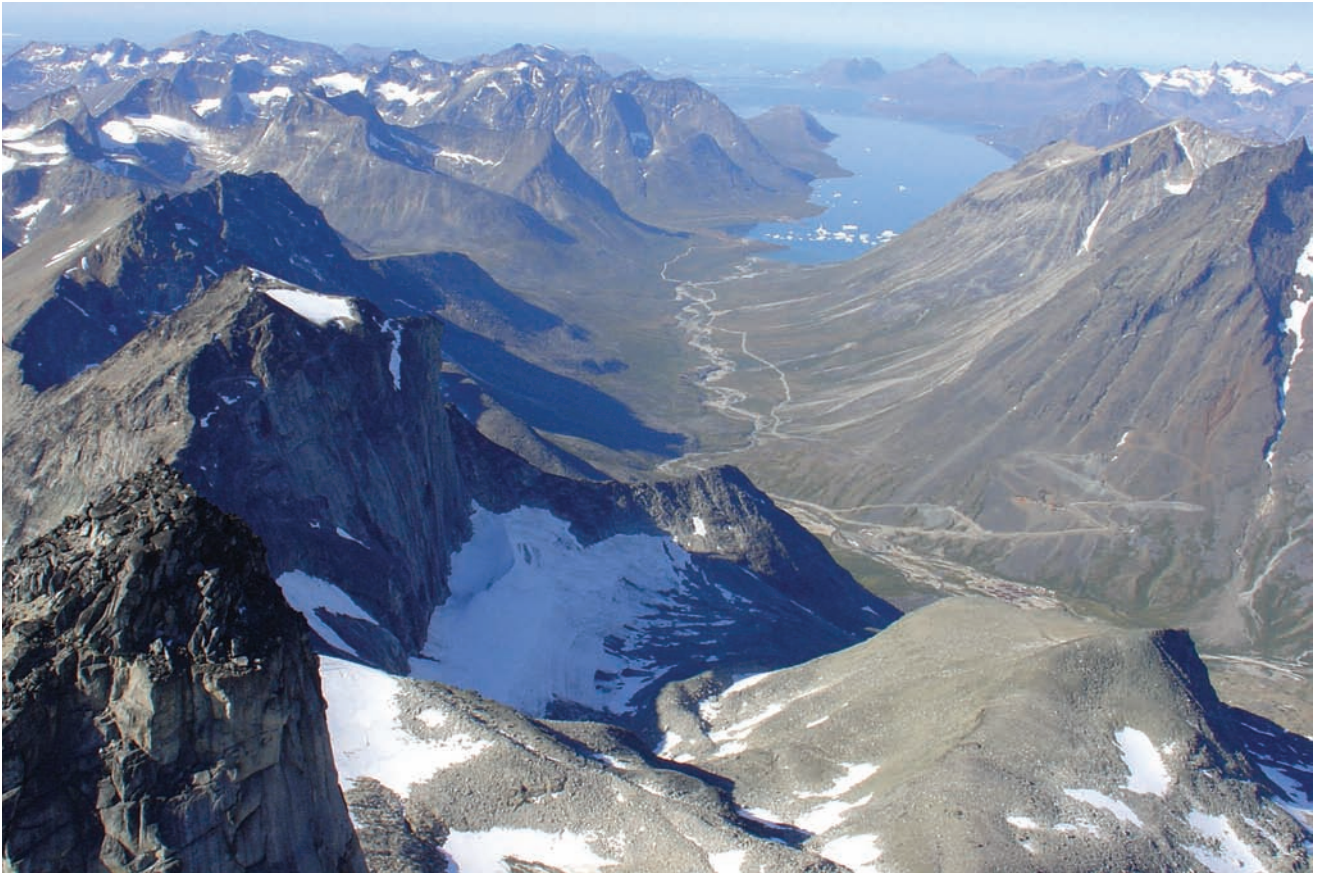
View westwards along the Nalunaq Gold Mine valley. The mine town and harbour road are situated in the valley floor. Mine roads on the mountain slope are connecting the three underground working levels (right).
